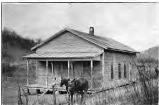
Four-Window Rural Schoolhouses, with Porch, but Without Cloakroom
